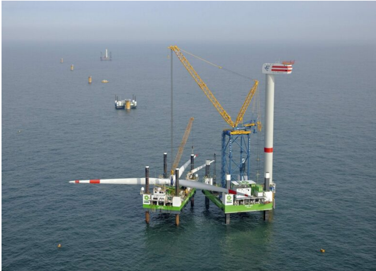
Offshore wind turbine installation.
